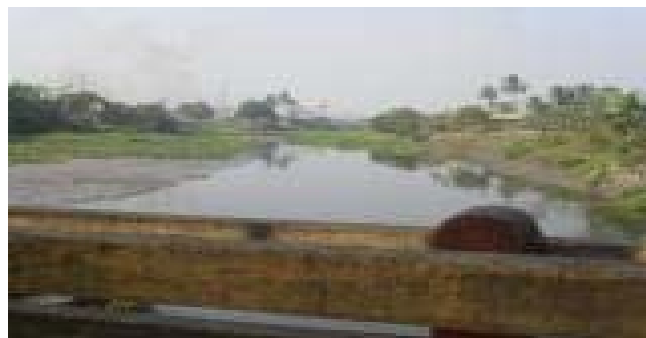
Fig. 5: The main DWF canal entering in the EKW area
